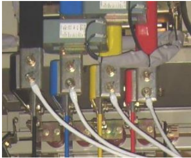
Connecting to R,S,T,N angular phase easy to install
